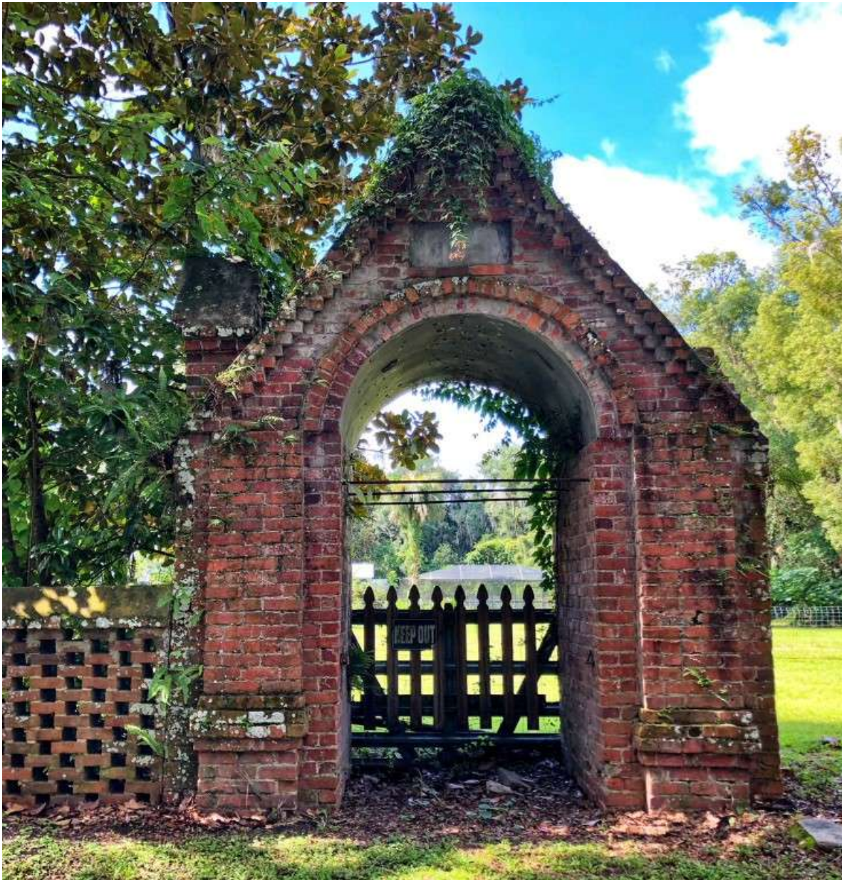
The Montgomery Wall in 2018. Photo: P Marlin
