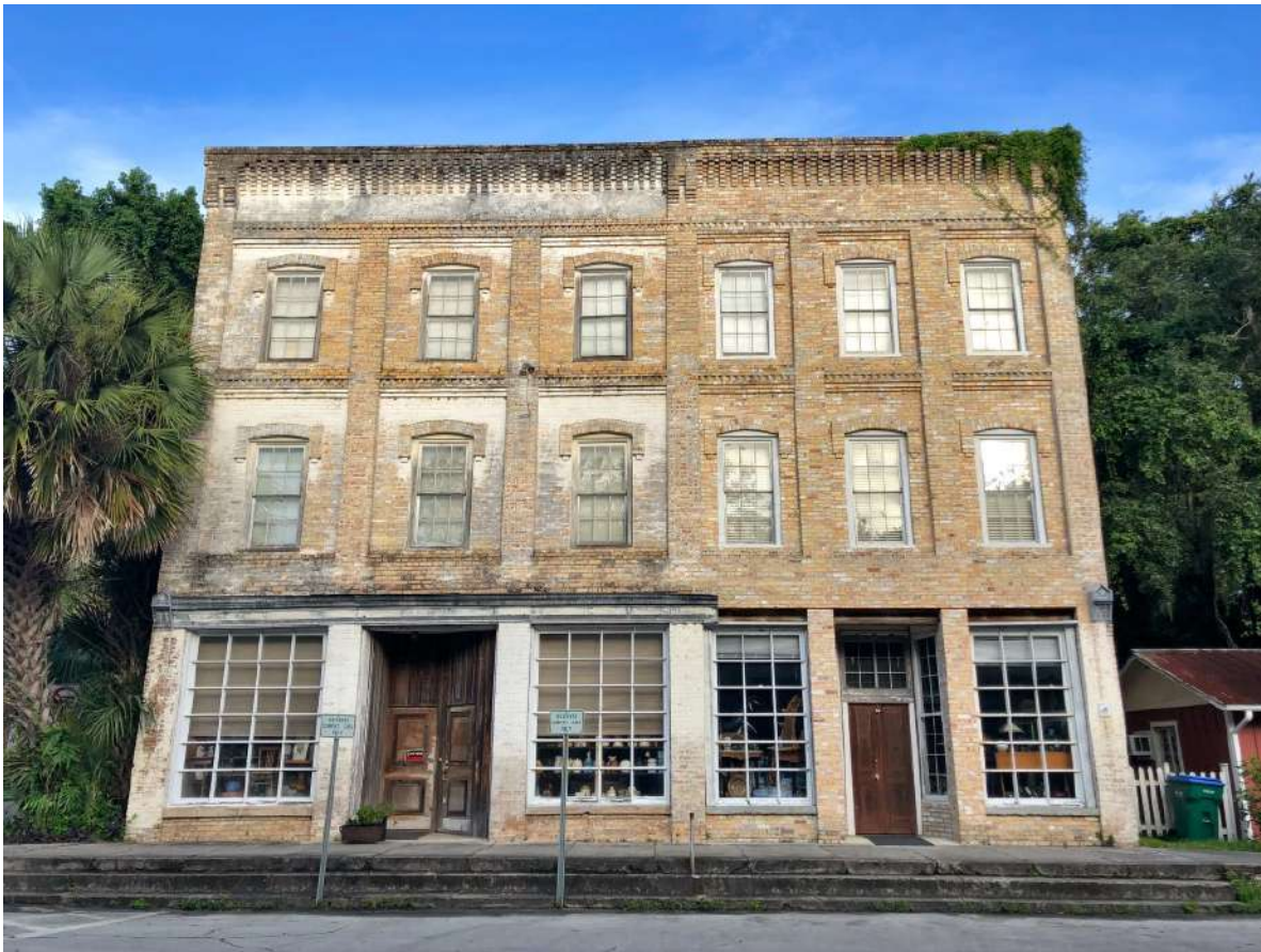
Feaster Building. Photo: P Marlin 2018
